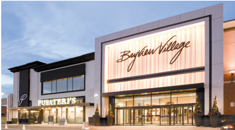
Bayview Village Shopping Centre
